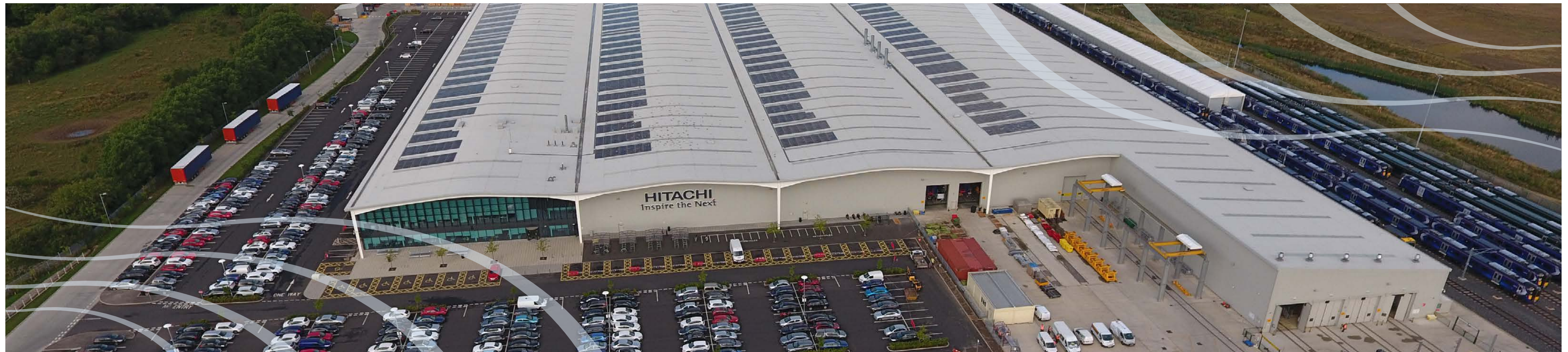
Newton Aycliffe Manufacturing Facility
