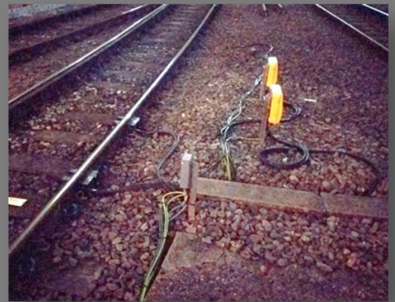
Figure 1: Example Redundant Detection Point Installation at Birmingham New Street
